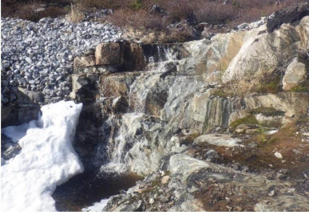
Photo 3.27 Lake F3298 outlet – View from downstream to upstream (April 2021)
