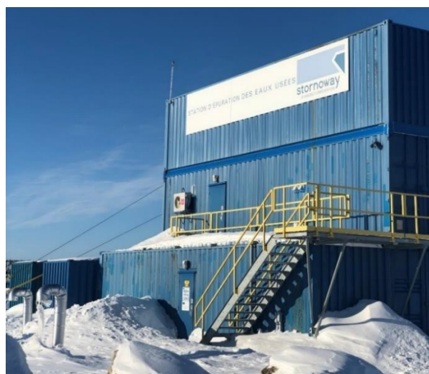
Photo 3.50 Domestic wastewater treatment plant (DWWTP)
