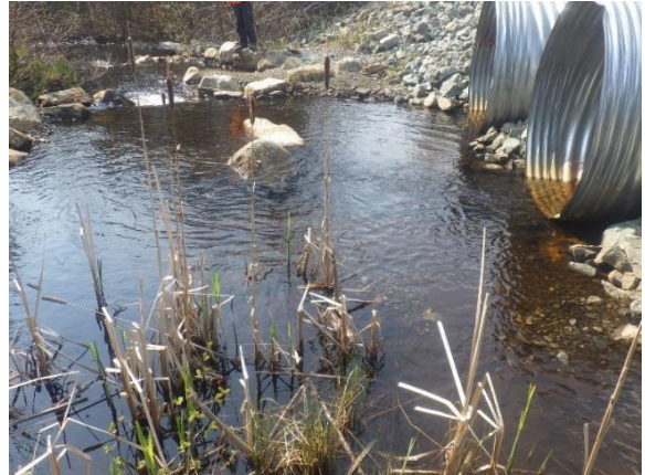
Photo 3.37 Spawning ground upstream from the culverts
