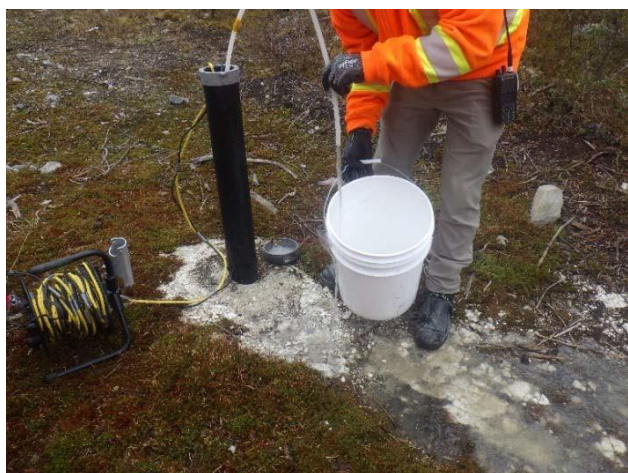
Photo 3.53 Groundwater sampling at the TLS (June 2021)
