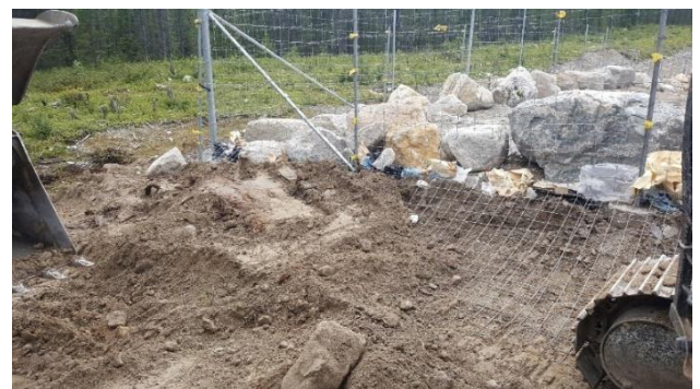
Photo 3.42 Reinforcing the fence at the TLS
