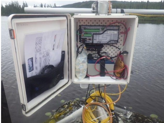
Photo 3.15 Inspection of the water level station at Lake F3300 in July 2021
