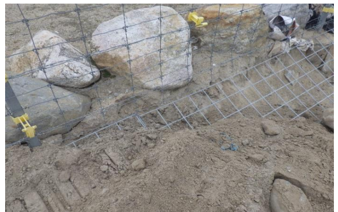
Photo 2.3 Installation of the fence around the TLS (June 2021)
