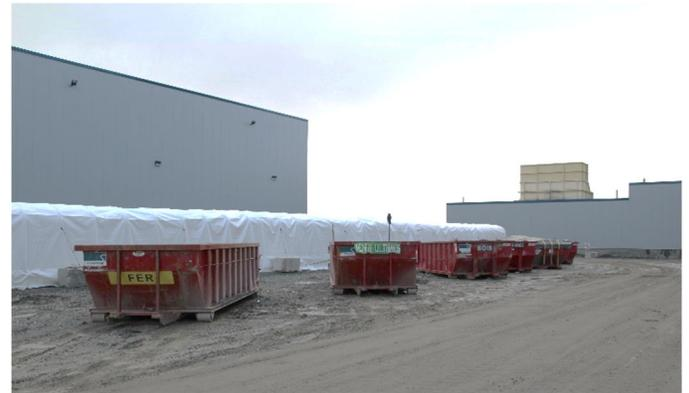
Photo 2.2 Source separation of residual materials on site
