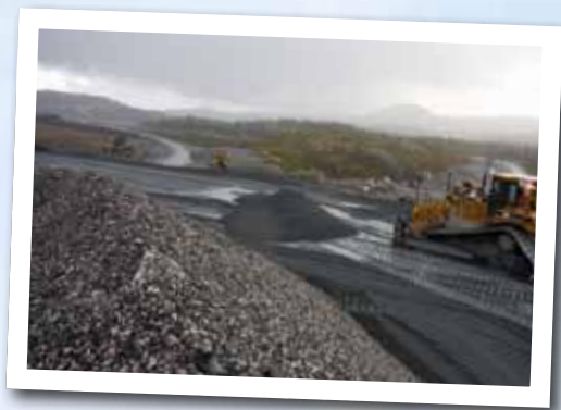
Construction of the permeable berm
