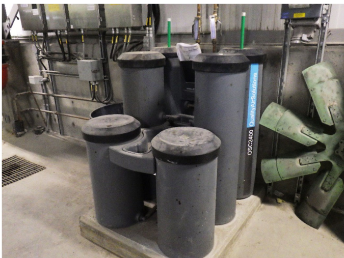
Photo 3.47 Fresh air (FAR) condensate separator
