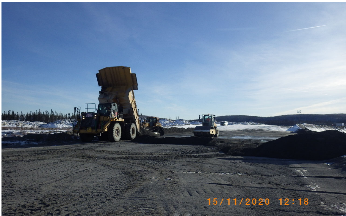
Photo 3.50 Deposition and compaction of processed kimberlite (coarse fraction) to raise a bearing downstream of the line center
