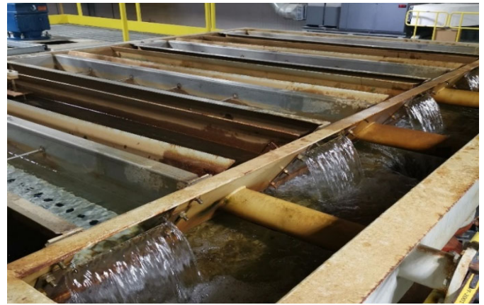
Photo 3.44 Treated water at the outlet to the lamellar clarifier
