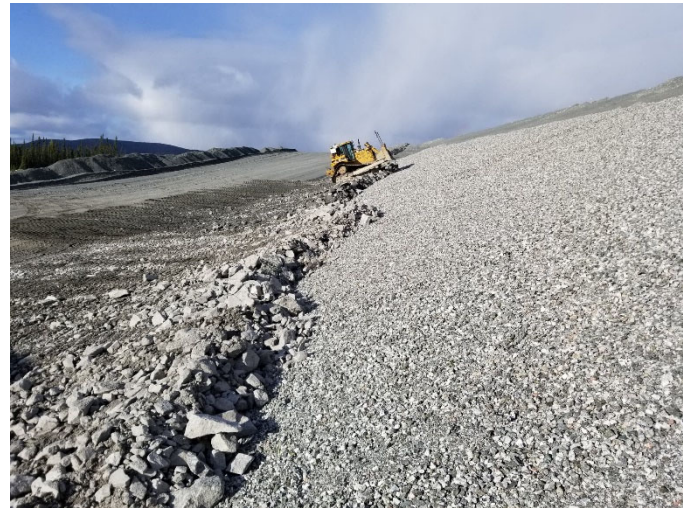
Photo 3.51 Installation of the stone layer for the progressive closure of the western slope
