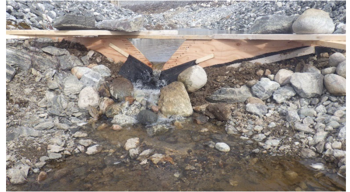
Photo 3.30 Graduated V-shaped weir in the lake outlet F3298
