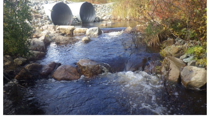
Photo 3.32 Weir built downstream of the culverts
